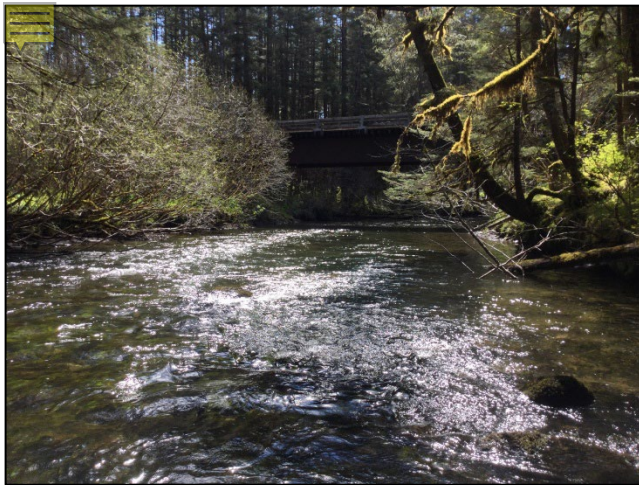
Figure 2.–Bridge at waypoint 111.
